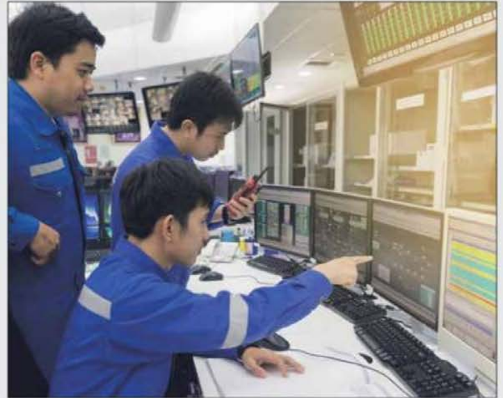
Operators in a metering control room for LNG.
