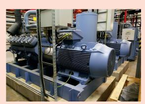
A two-stage screw, or reciprocating, compressor with interstage and second stage cooling is the ideal compressor configuration in an ammonia chilled CO2 liquefier. In a 4 tonne per hour liquefier an ammonia compressor of circa 350 kW could be suitable. This increases to around 600 kW for a 7 tonne per hour CO2 liquefier. Ammonia is compressed to around 15 bar in the chiller refrigeration cycle.
