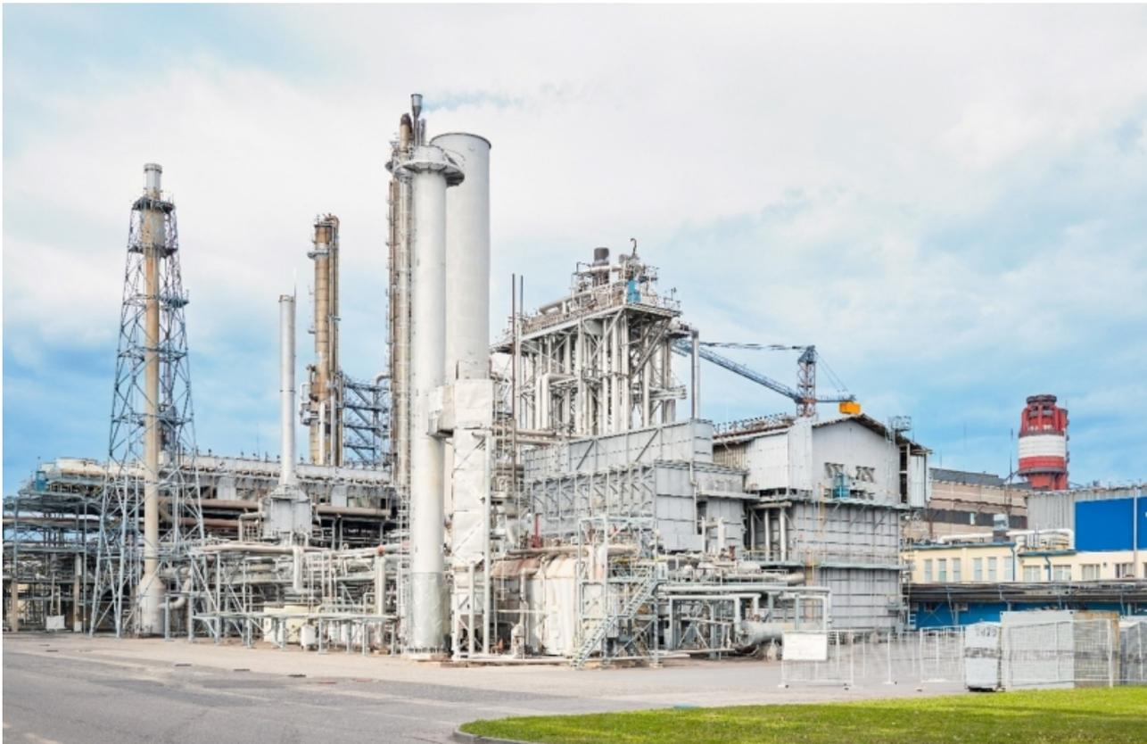
Steam methane reformers consume natural gas to make grey hydrogen and they emit carbon dioxide as a consequence. In the long term, that can be mitigated with a transition to 'green' hydrogen production using electrolyzers which can be fed with renewable electrical power or steam methane reformers fed with renewable biogas.
