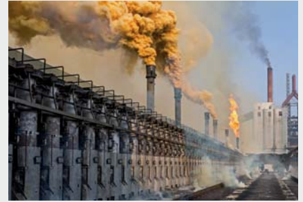
Raw flue gases that are rich in CO can be utilized to produce ethanol in a bioreactor. Ethanol can be used for many chemical and energy applications.
