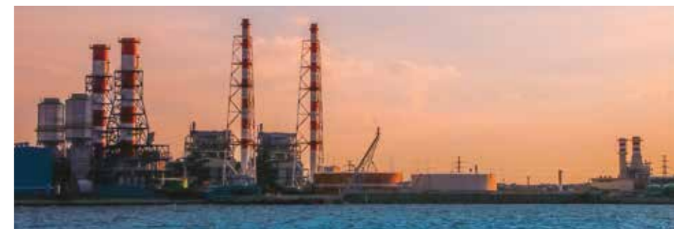
Gas fired power plant, Jakarta, Indonesia
