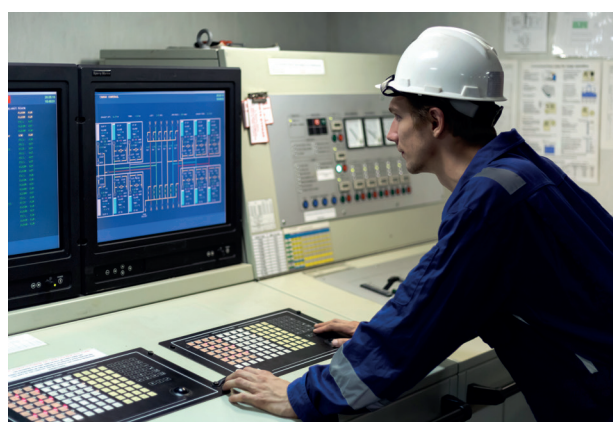
Cargo hold monitoring system
