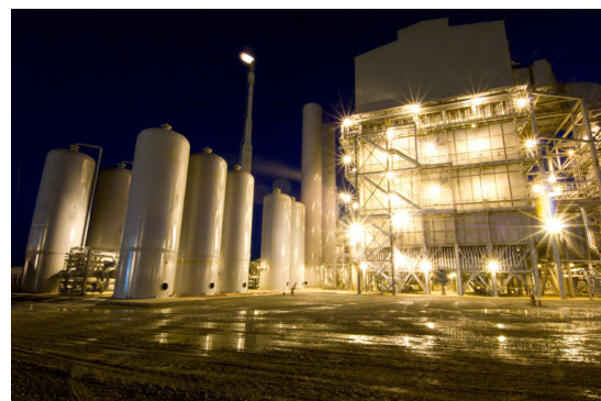
Source: Air Products SMR Convent Louisiana
