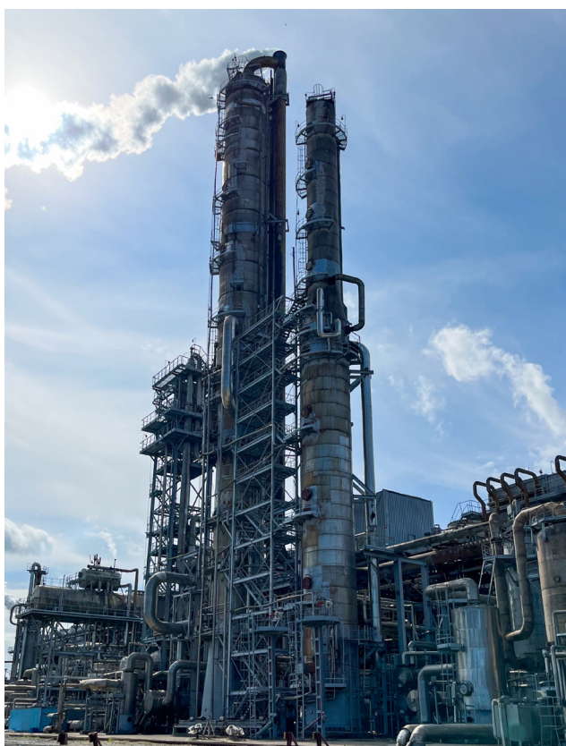
Figure 4. CO 2 absorber and stripper on ammonia plant.
