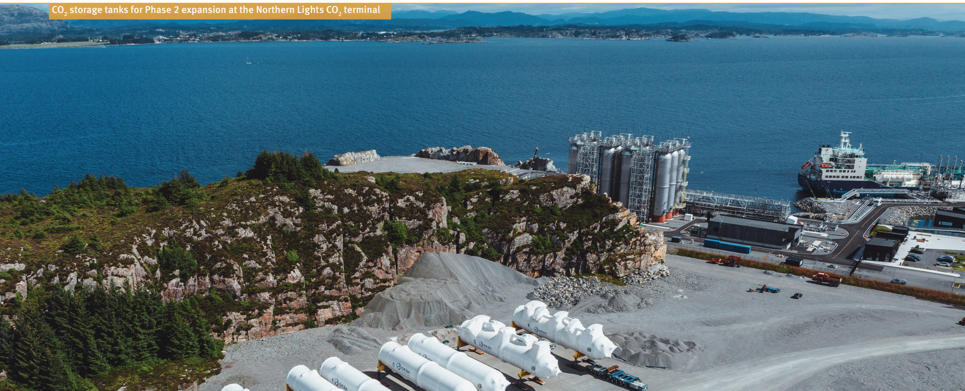
CO 2 storage tanks for Phase 2 expansion at the Northern Lights CO 2 terminal
