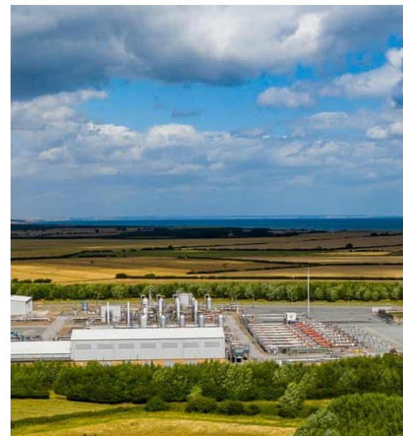
UHS to be implemented at an existing SSE site in Aldbrough on the Yorkshire coast in the UK.
