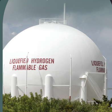
Liquid hydrogen sphere Kennedy Space Centre Cape Canaveral
