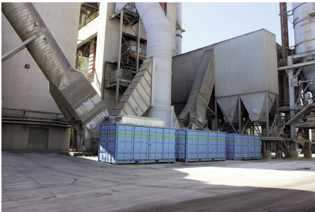
Chart's Cryogenic Carbon Capture process (CCC) exploits the gas to solid deposition phase change that is unique to CO 2 . Image: ©Chart Inc
