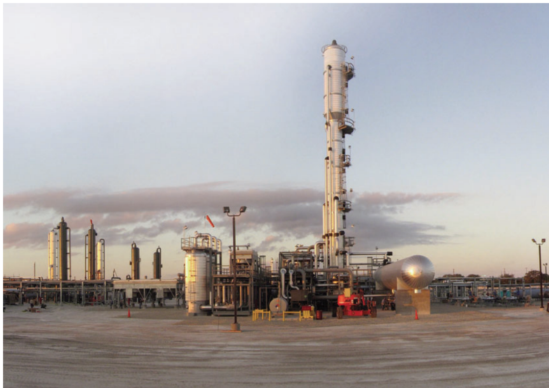
The Orloff process owned by Honeywell yields very pure CO 2 and operates in a manner which prevents solid CO 2 formation. Image: ©Honeywell UOP
